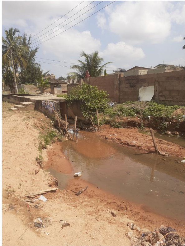
Fig. 7 Road erosion caused by partial drainage from uphill areas in Santa Maria. Source: authors' fieldwork, 2019
