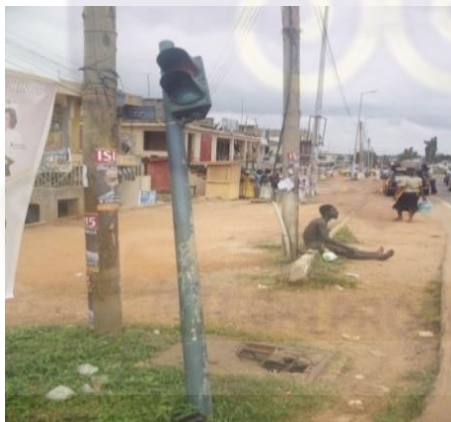
Plate 9: Non-Functional Traffic Light at Pipe (Tanokrom) Circle
