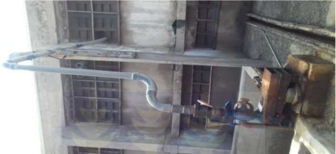
Figure 3.1. 4: A filtrating pump for transferring separated salt from the centrifuge cell into a classifier.
