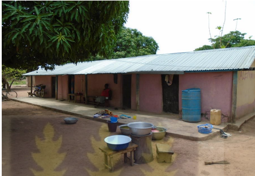
Figure 5.7: A four-bedroom infrastructure serving as wards for patients in the Papakesie shrine. Picture taken by the researcher at Ehiamankylene, Krachi West Municipal. 23 rd March, 2021.
