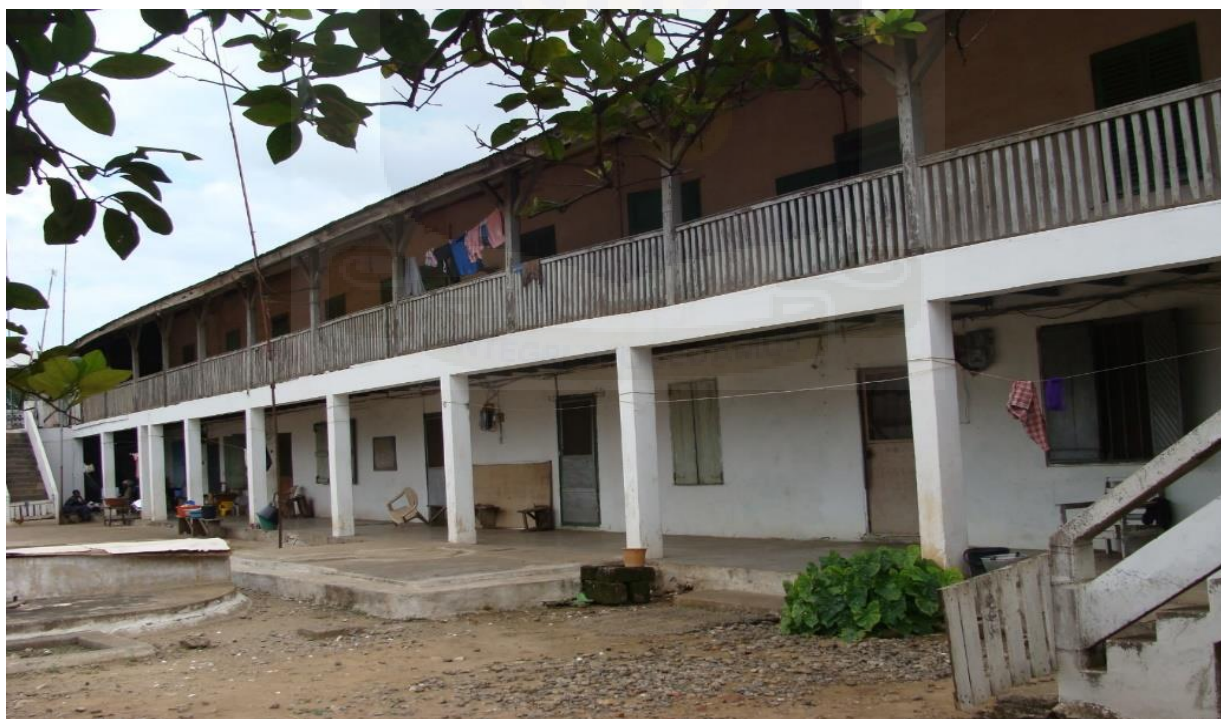
Figure 17: Residential unit at the UTC yard (source: Gideon Agyari)
