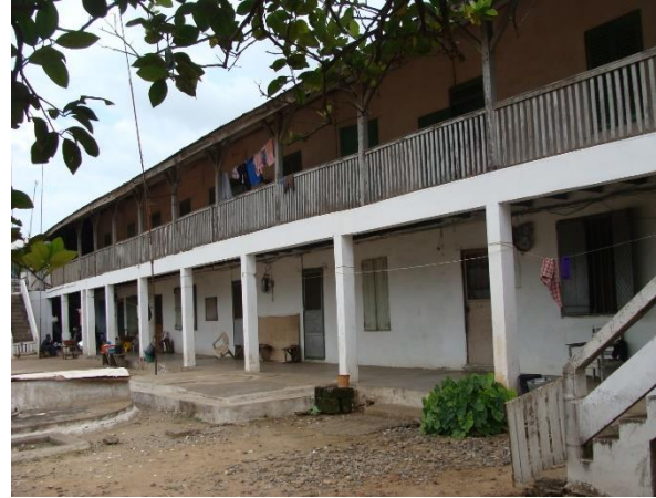
Figure 6: abandoned UTC warehouse
