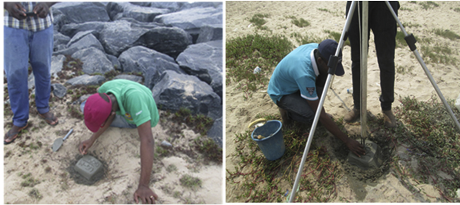
Fig. 2. Establishment of control points.
