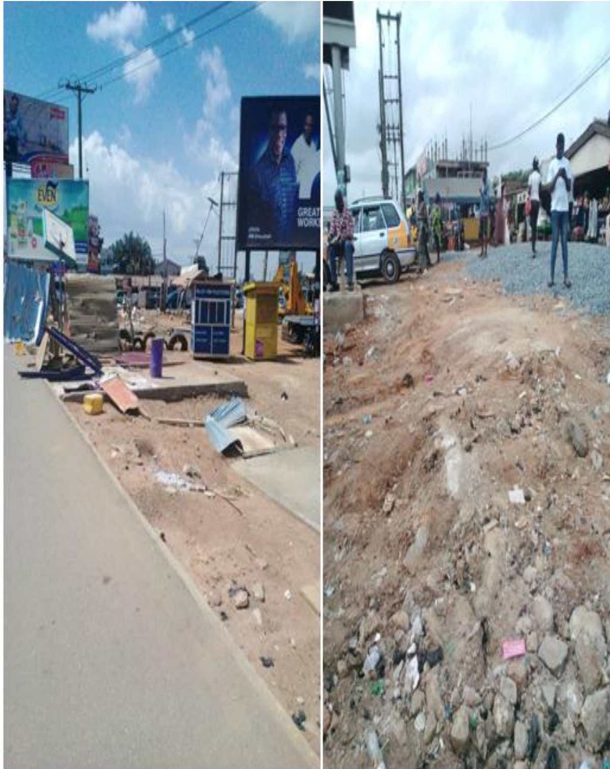
Figure 6.4 some newly demolished areas after decongestion exercise
