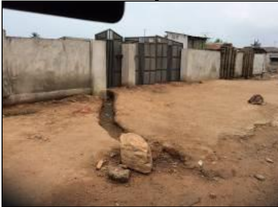
Plate 7.1: Earth Drain –Mpoase
