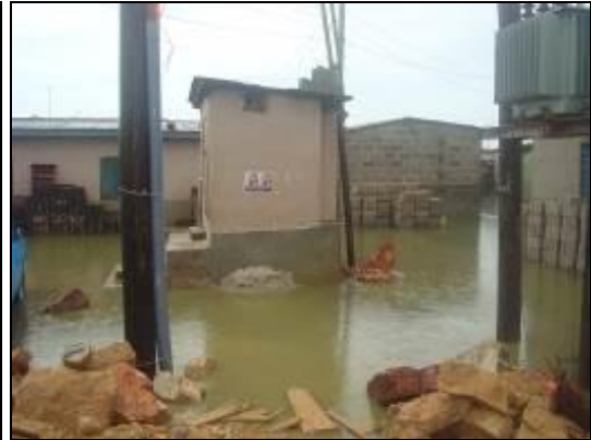
Plate 7.2 Toilet with a Raised Foundation-Glefe
