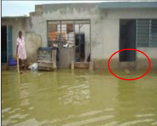
Plate 7.3: Raised Door Step-Mpoase
