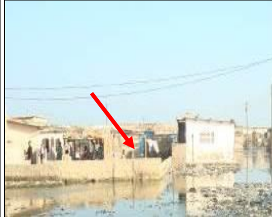
Plate 7.4: Building with a Retaining Wall-Glefe
