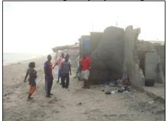
Plate 1.4: Building Destroyed by Storm Surge-Glefe
