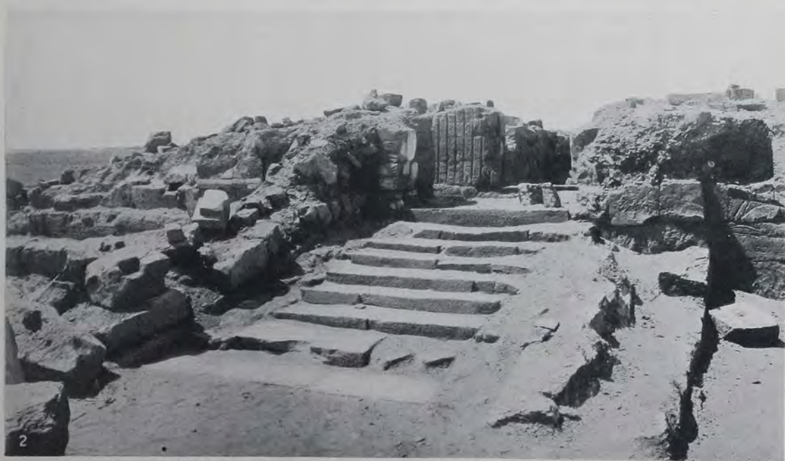
1. View from NE. after excavation, showing the entrance (1).
