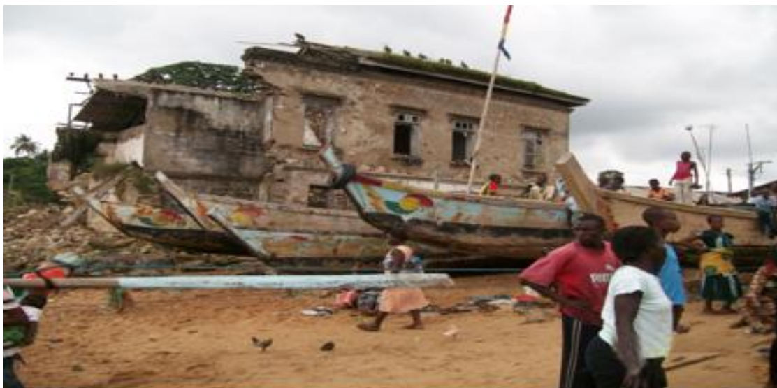
Plate 8.5. One of several European architectural styled houses which were owned by wealthy Indigenous merchants sited close to the beachfront (Picture: Fritz Biveridge)
