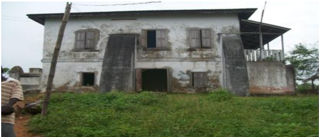
Plate 8.2. This storied structure is the oldest church to be established at Dixcove. An epitaph on the extreme lower left corner dates the structure to April, 1856 (Picture: Fritz Biveridge).
