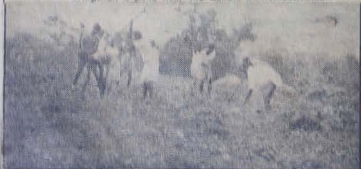
VOLUNTARY WORKERS at work on a new road.
