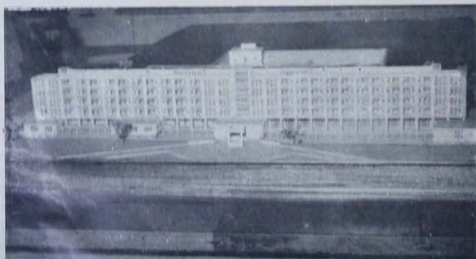
A MODEL of the Accra Hotel. Work on the building goes on day and night.
