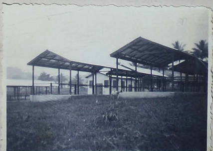
A New Market under construction.
