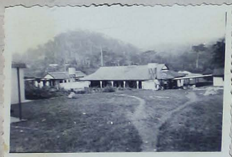
A Section of the Kibi Hospital.
