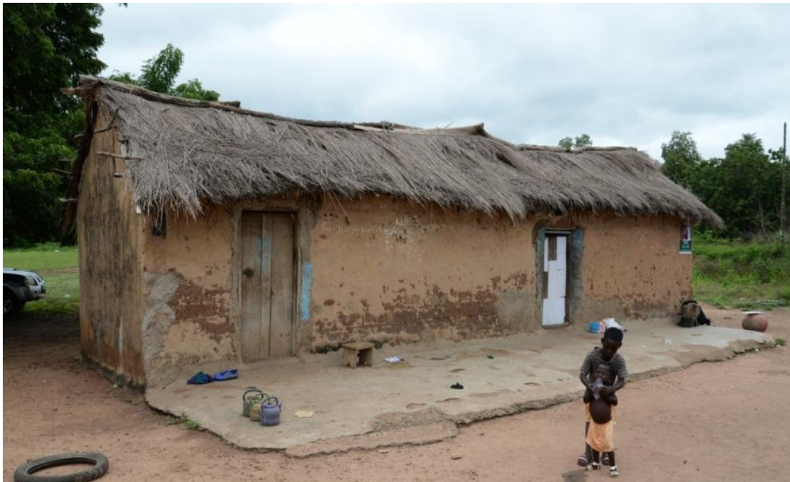
Fig. 4.2: Rectangular mud-brick structure with saddleback triangular truss thatch roof (by D. Genequand, 2016)
