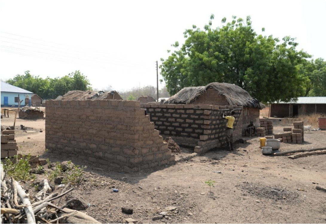
Fig. 4.9: Raising the mud-brick wall of a house (Photo by D. Genequand, 2017)
