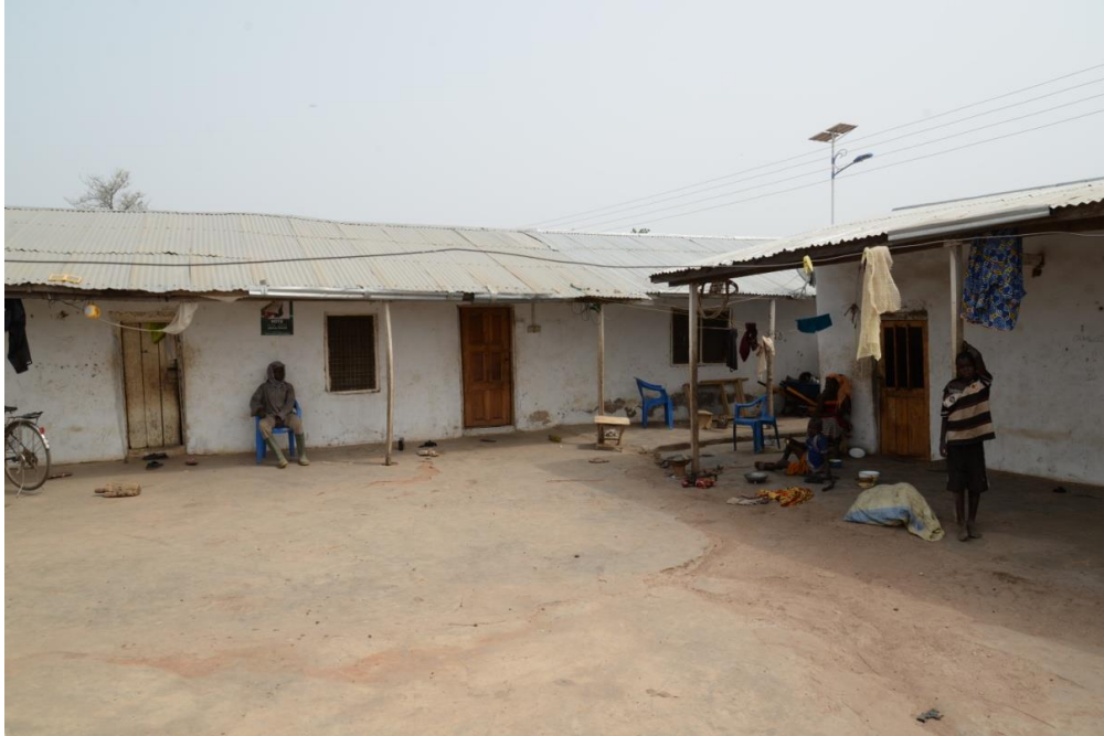
Plate 7: Aluminium/zinc roof and cement plastered courtyard of a compound (by D. Genequand)
