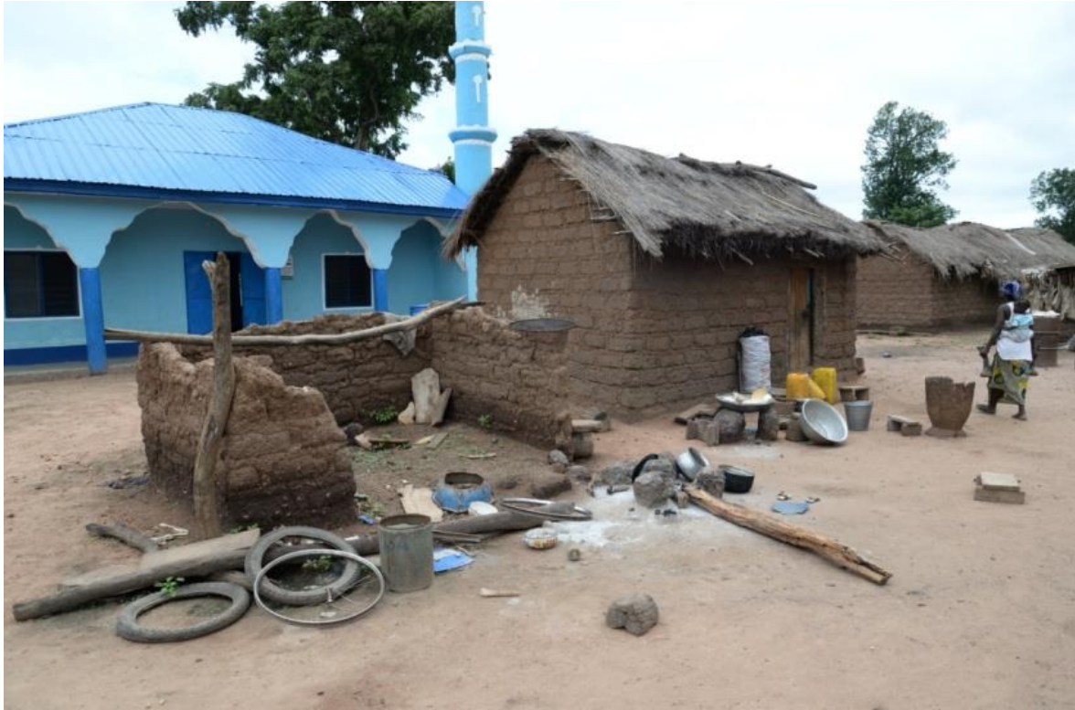
Fig. 5.6b: A collapsed and a newly constructed adesikpa (by D. Genequand)
