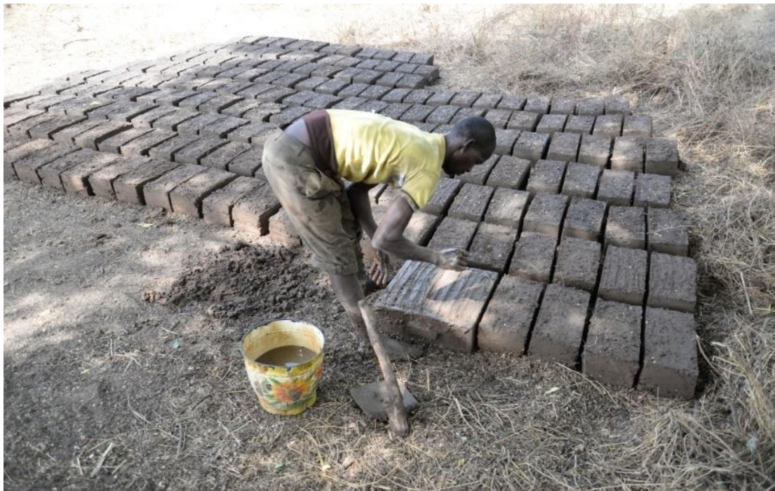
Fig. 4.8: Grooving in mud during brick making process (Photo by D. Genequand, 2017)
