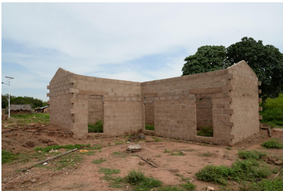
Fig. 5.11: Modern building type with industrial materials (Photo by D. Genequand)
