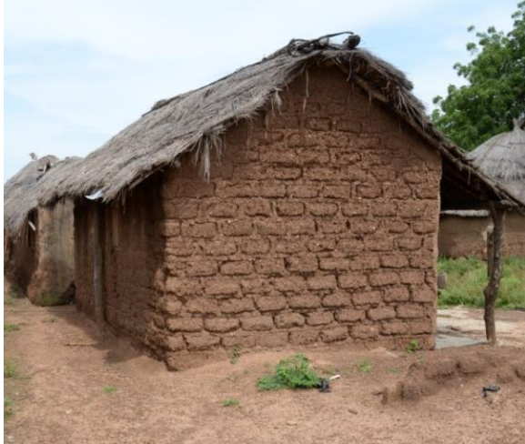
Fig. 4.16: Triangular truss roofing style on gable walls (Photo by D. Genequand)
