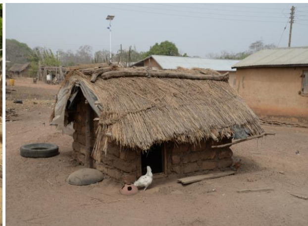
Fig.5.7b: Rectangular-shaped mud-brick coop/pen
