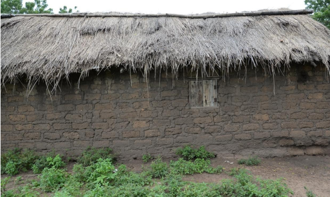
Fig. 5.14: Fragments of ceramic in the fabric of mud-brick wall (Photo by D. Genequand)
