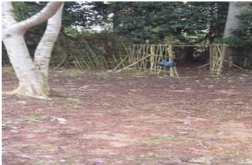
Figure 18 Construction of Entrance Source: Researcher, fieldwork, 28/02/2016
