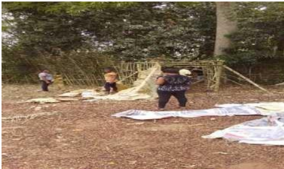
Figure 19 Covering of Entrance with jute and cement papers Source: Researcher, fieldwork, 3/03/ 2016
