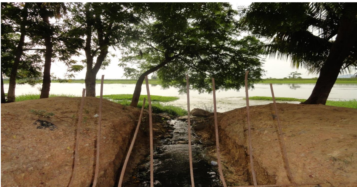
Plate 2 A sewage draining into the Kpong reservoir
