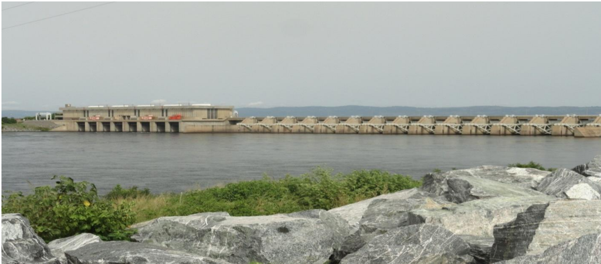
Plate 1 A cross section of the Kpong dam showing a section of the Reservoir
