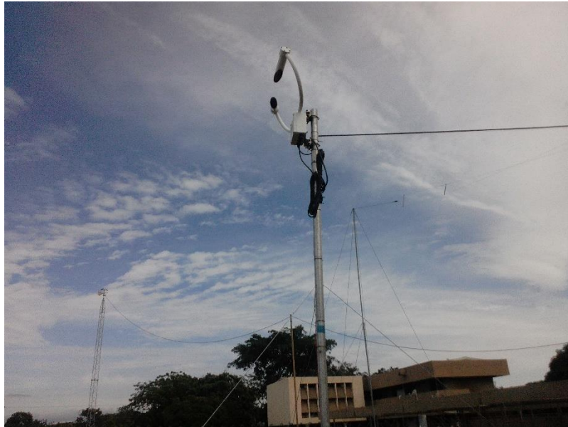
Figure 4.16: Fully mounted visibility sensor
