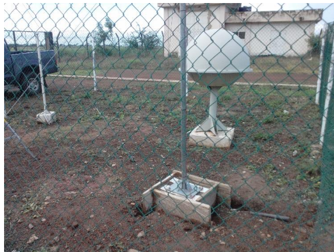
Figure 4.15: Concrete foundation for mount installation
