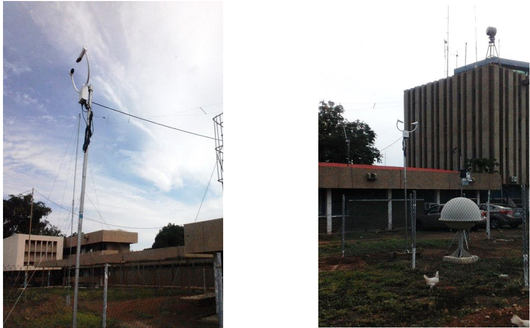
Figure 4.16: Set up the CS120 Visibility Sensor and Vantage Pro 2 Weather Station at the Tamale site
