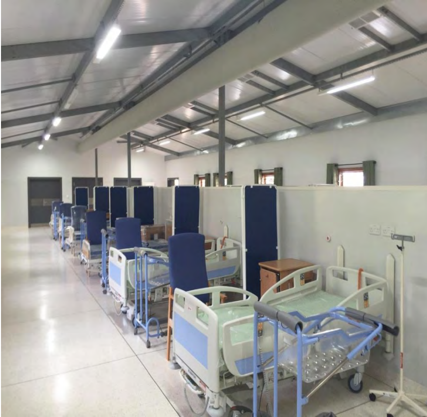
Figure 4: A Typical Ward in Shai-Osudoku District Hospital
