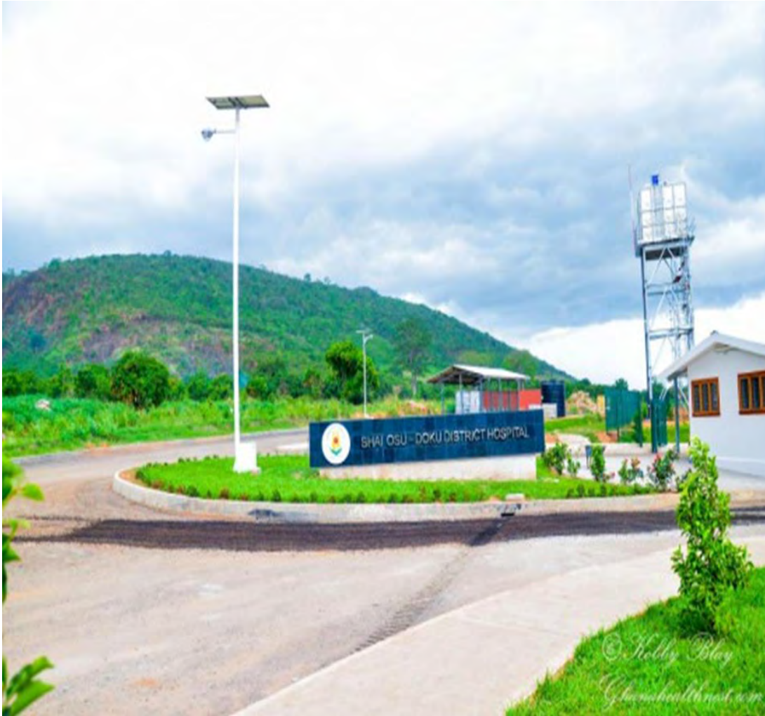
Figure 2: Shai-Osudoku District Hospital
