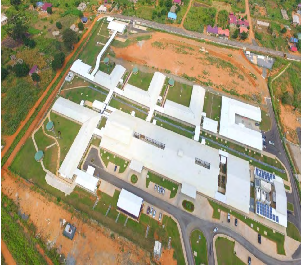
Figure 3: Aerial View of Shai-Osudoku District Hospital
