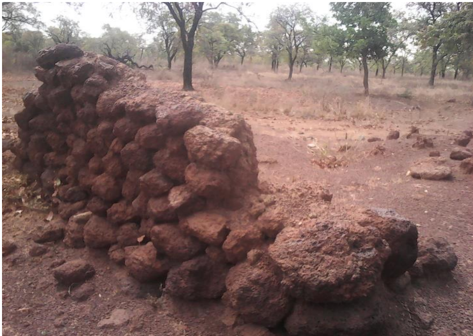
Fig. 26: Remains of an abandoned house at Pizaga (Photo by J. Ampofo Manu, 2019)
