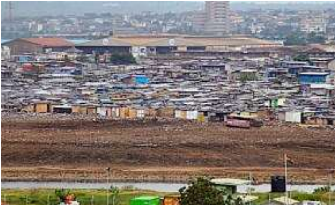
Figure 3.1: Housing Structures at Old-Fadama
