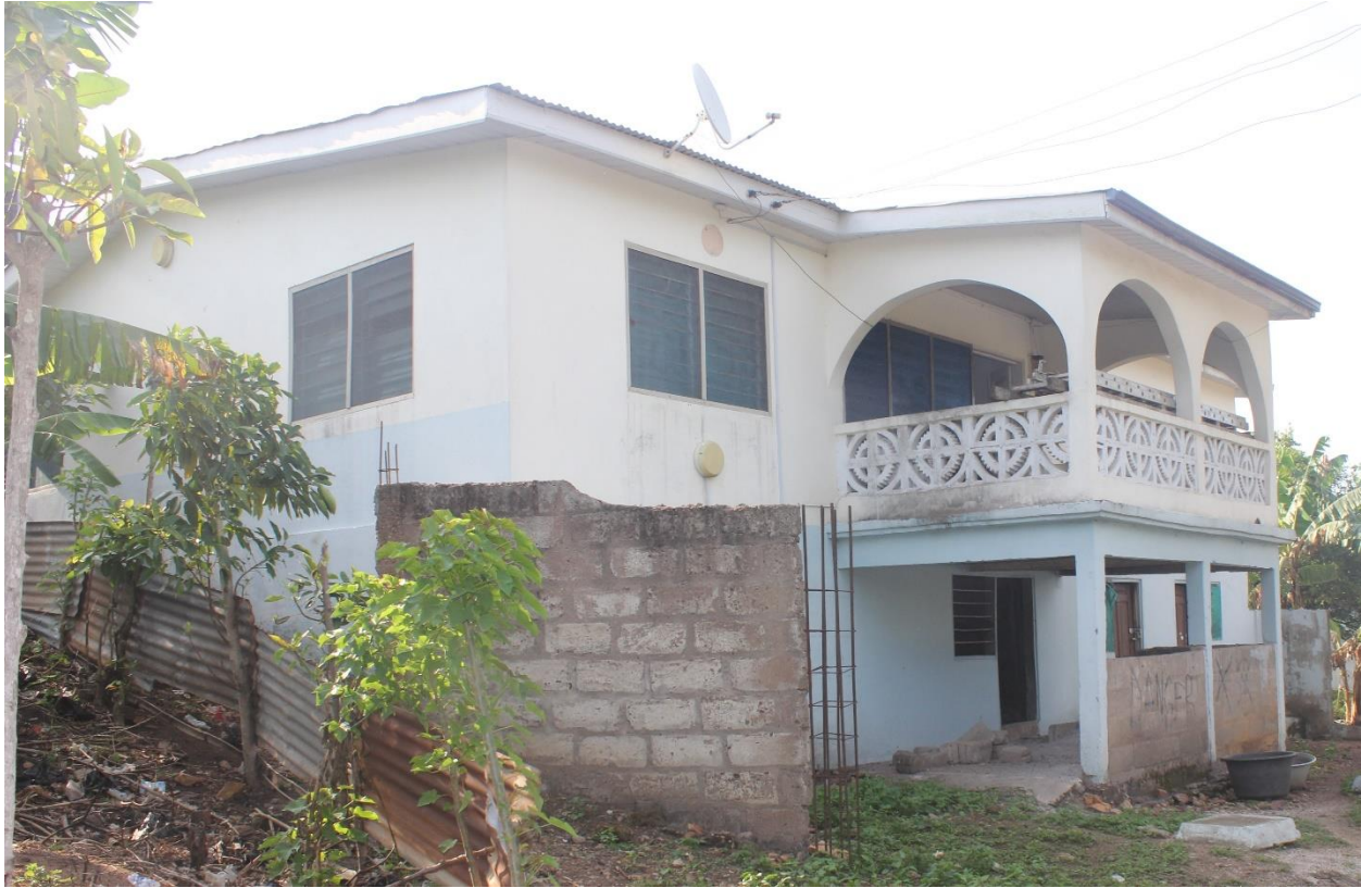
Figure 3.4 Picture of a house built with cement and blocks at Larteh. (Photo credit: Author's collections).
