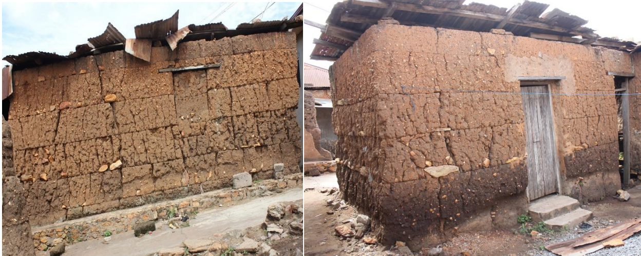
Figure 3.2 Picture of wattle-and-daub structures at Larteh. (Photo credit: Author's collections).
