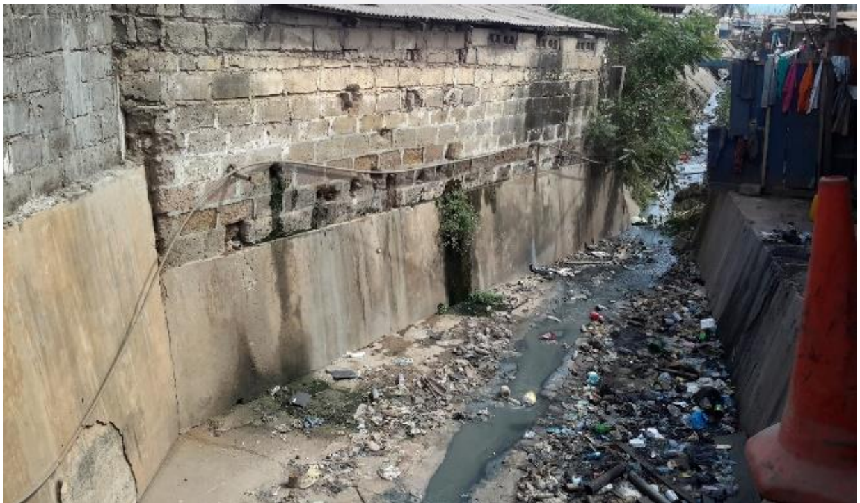
Plate 3. 2 Pipelines found in drains in La
