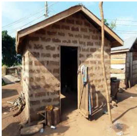
Plate 3.2: Cement kitchen with zinc roof
