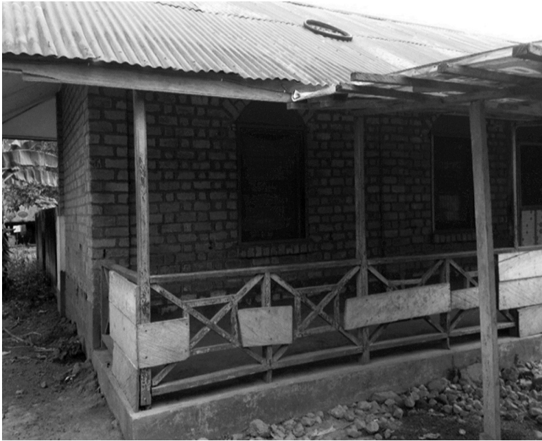
Figure 4.1 An experimental swish building for the Forestry Commission at Kibi, built in the 1950s (Iain Jackson, 2018; reproduced with the permission of Prof. Jackson).
