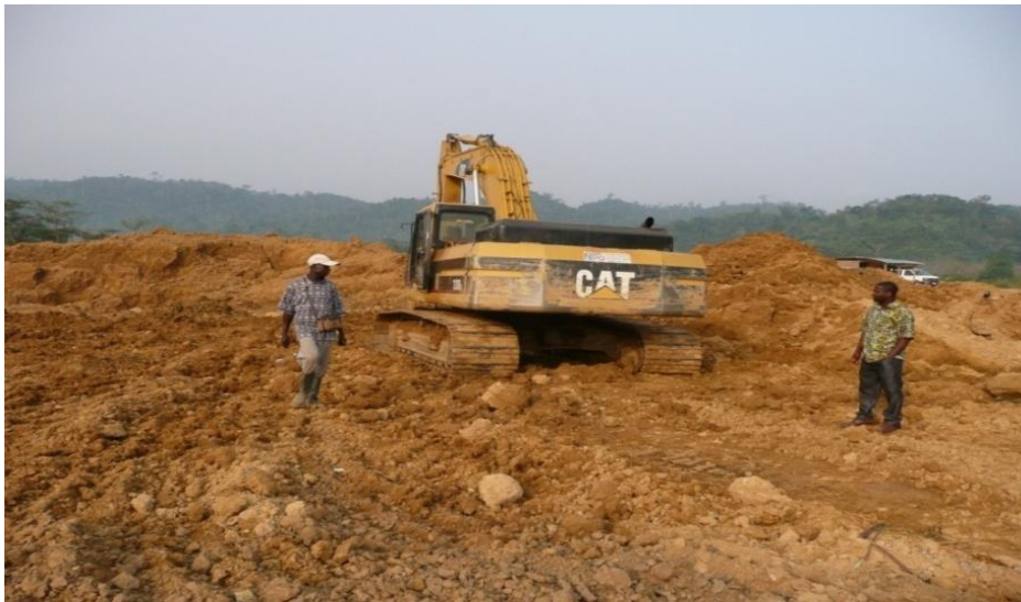
Plate 3: An Excavator Degrading Land during Surface Mining
