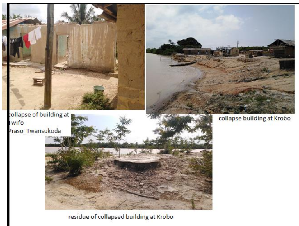
Figure 6.2: Field pictures showing residues and collapse building
