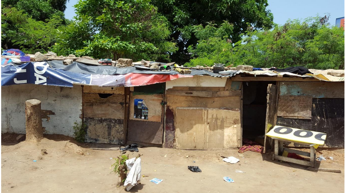
Figure 4.2: Exterior view of wooden structure.
