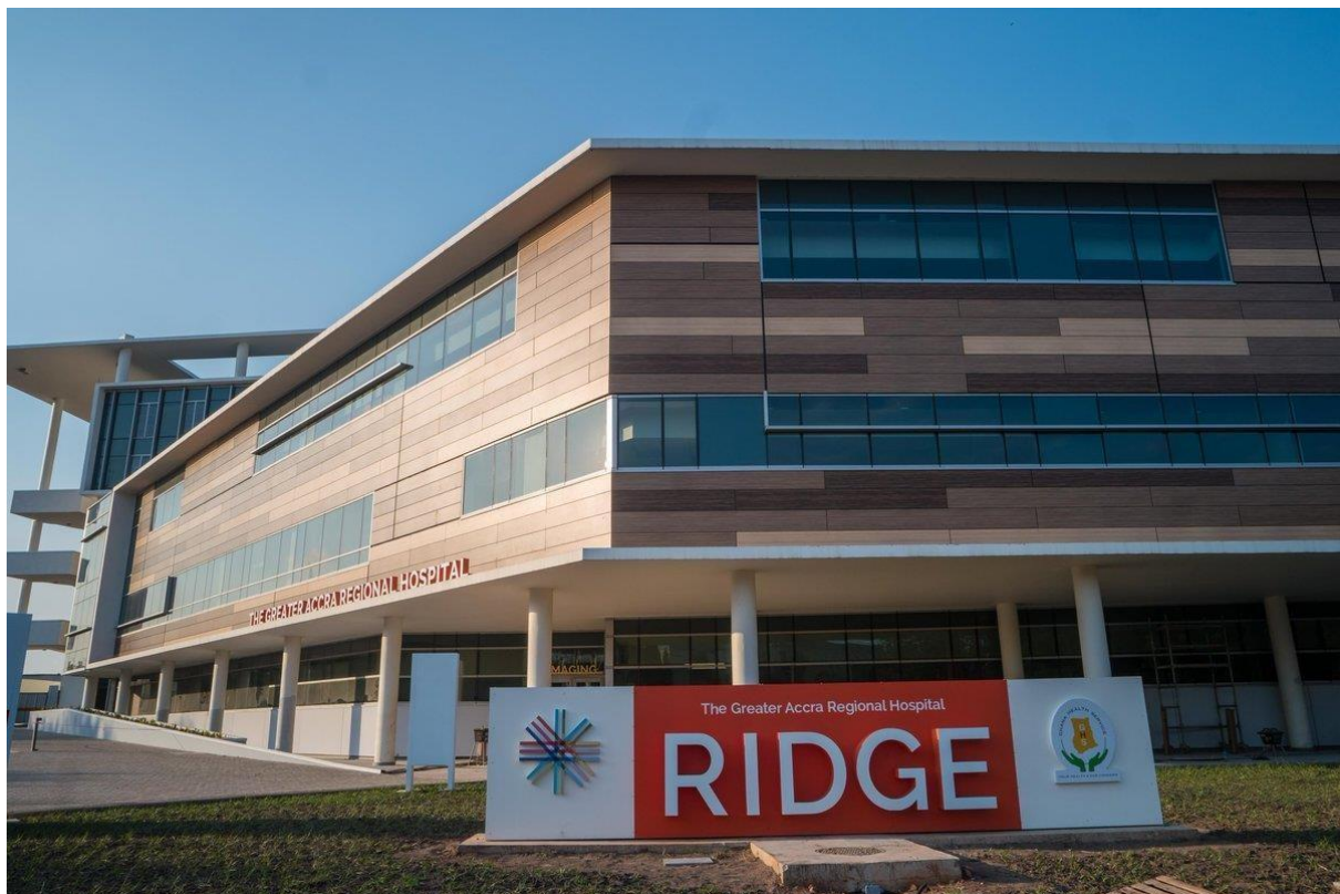
Figure 4: Picture of the Greater Accra (Ridge) Regional Hospital
