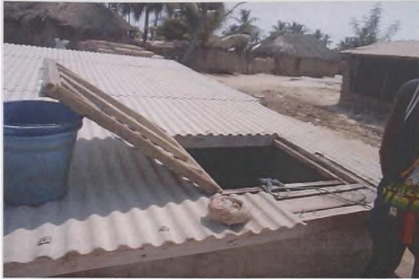
Fig. 21. Tank with complete cover (sloped)
