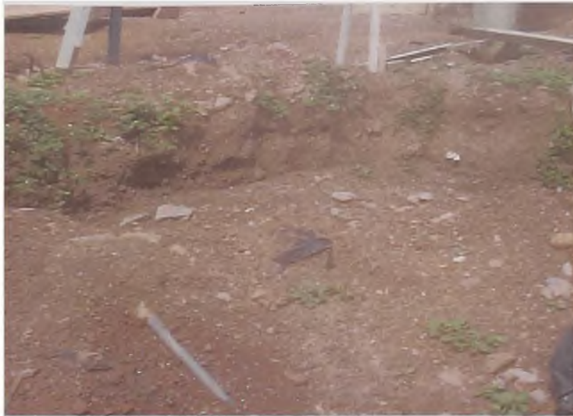
Fig. 8. Contamination of chlorinated water through leakages
