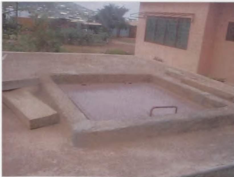
Fig. 22. Tank with complete cover (not sloped)
