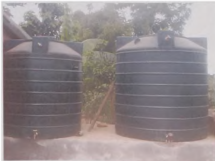
Fig. 20. Poly tanks above ground with tap outlet
