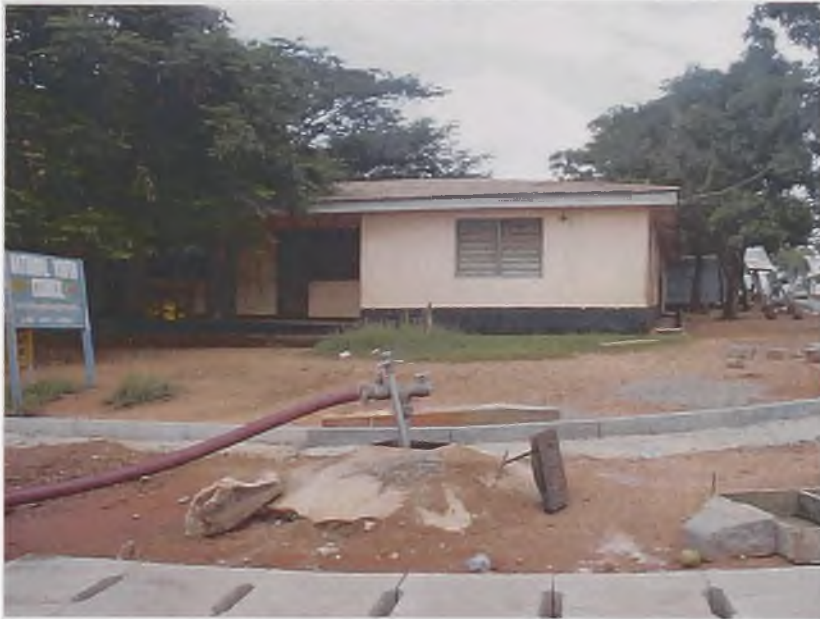
Fig. 6. Contamination of chlorinated water at hydrant
