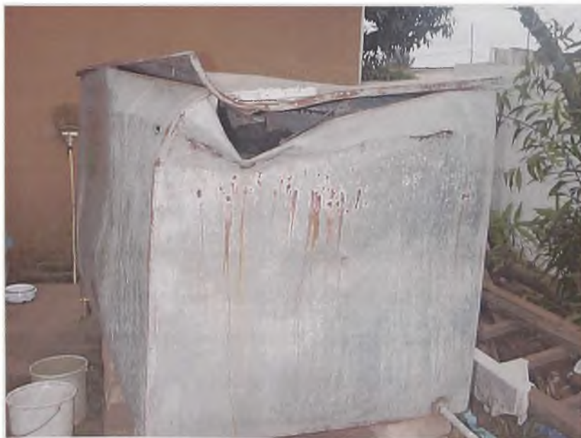
Fig. 9. Contamination of chlorinated water through defective reservoirs and tanks
