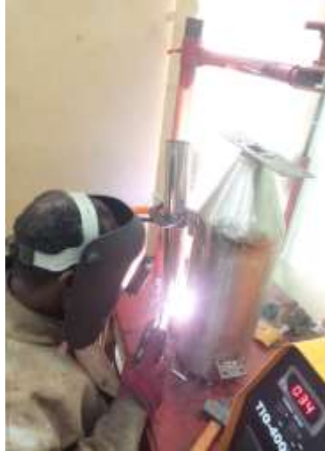
Figure 3.8: Welding of parts together
