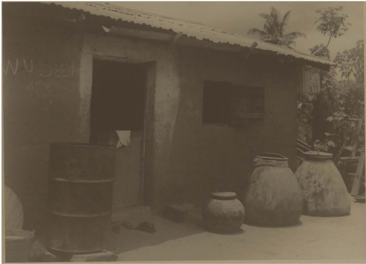
Plate 8: A mud house at Amasaman showing the different types of water receptacles. The guttering allows rain water to fall directly into the jars during a rain storm.
