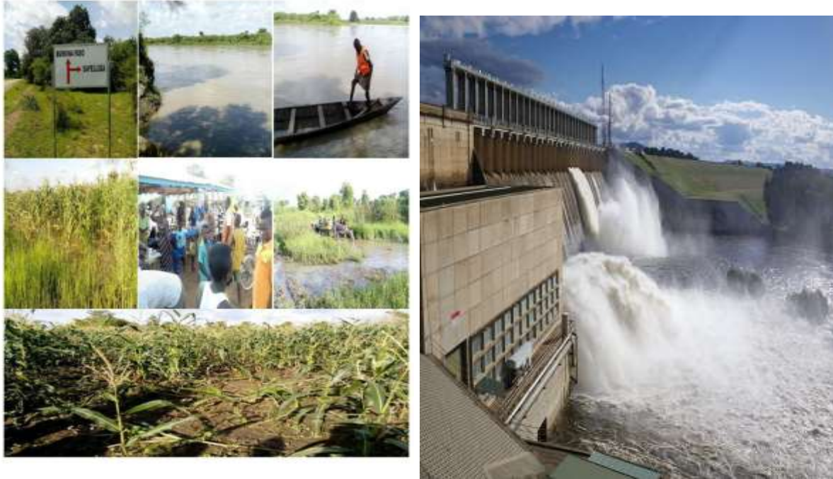
Figure 2.5 Bagre Dam Spillage, 2019
