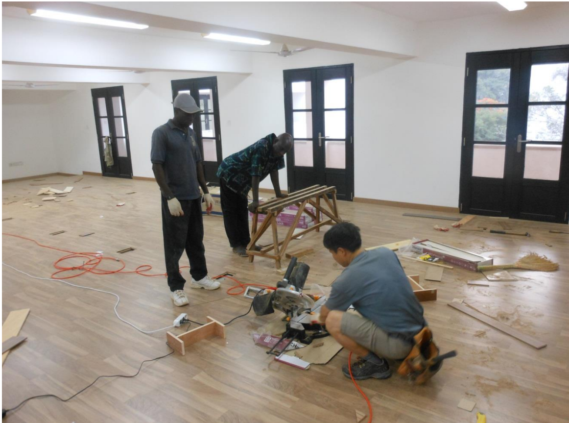
Figure 6- Information Access Center under construction
