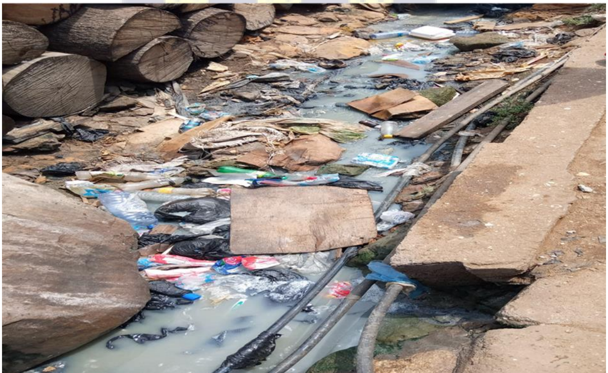
Figure 4.10: Garbage disposed into open drain with water pipelines in Chorkor, Accra
