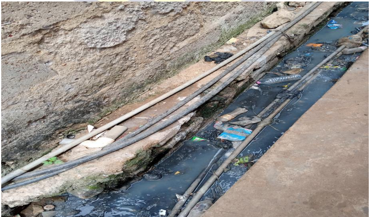
Figure 4.17: Garbage disposed into open drain with water pipelines in Nima, Accra
