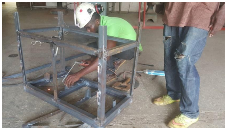
Figure 4.6: Welding Main Frame of the Improved Cook stove
