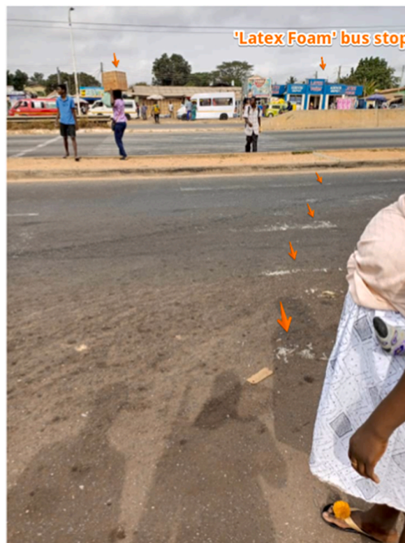
Fig. 3. Pedestrians taking the risk of using the informal crossing (one with a piece of head luggage) despite its faded, marked stripes.
