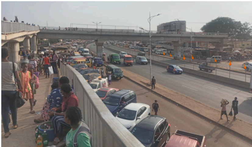
Fig. 5. Wire mesh used as road safety barrier (arrowed red) at the Redco Junction Footbridge .
