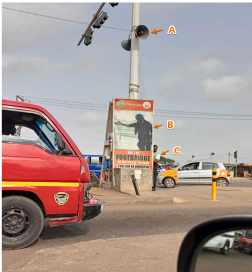
Fig. 6. Pedestrian safety measures (Note: Audio (A) and visual (B) warnings together with a City Guard (C) to enforce pedestrian) adopted near the Zongo Junction Footbridge.
