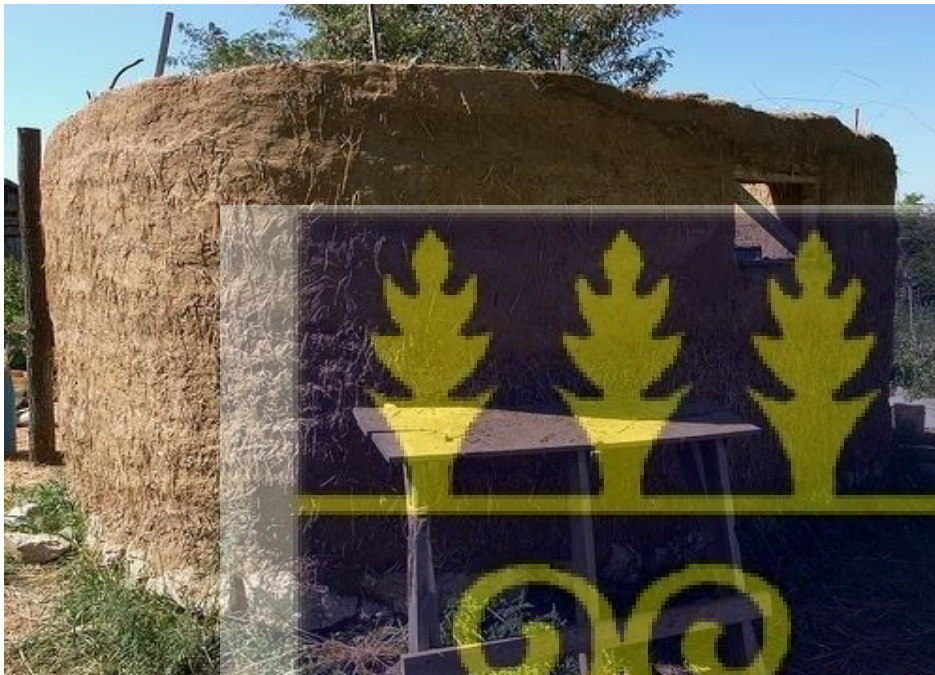
Figure 2. 3 Cob structure (Danso, 2016)
