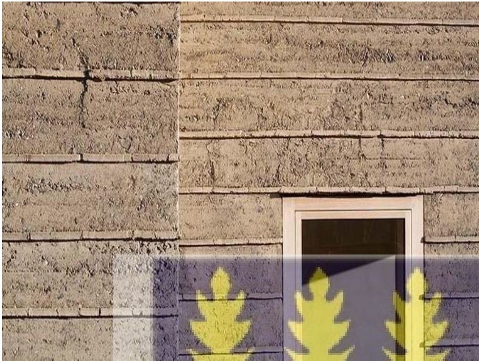
Figure 2. 4 Rammed earth (Danso, 2016)
