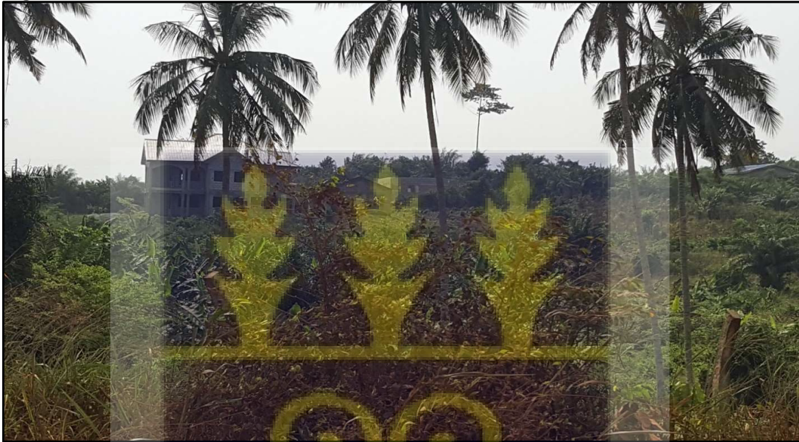
Figure 5.5: House under construction in PuMI Mampong, which is situated amid vegetation. An indication of farmlands being converted to residential use
