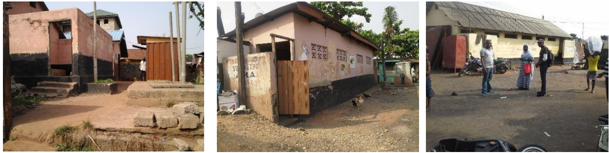
Plate 5.5 Public toilets in Maamobi-Nima
