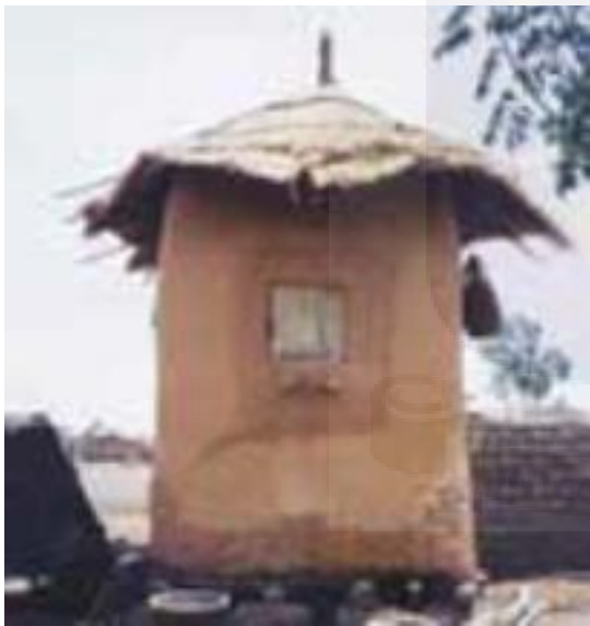
Plate 2.9: Mud storage structure
