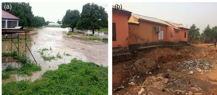
Figure 4. During and following flooding event in the study communities.
