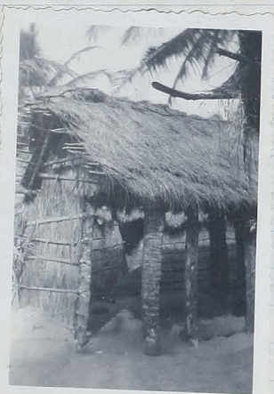
A HAMLET IN BUILDING AT FA NA FISHING VILLAGE SHOWING THE WALL WITH WOODFRAME AND GRASS
