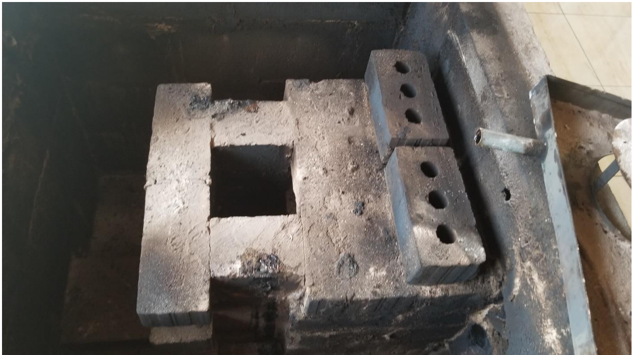
Figure 2.3 Internal view of “Ahotor” oven showing combustion chamber made of sandcrete blocks.
