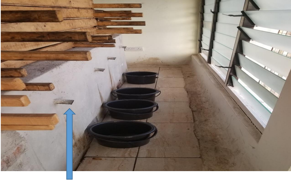
Figure 2.4 Fat exit of “Ahotor” oven.
