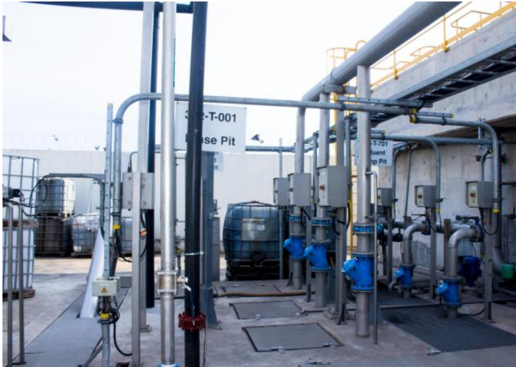
Figure 4.2.6 The Effluent Pit
