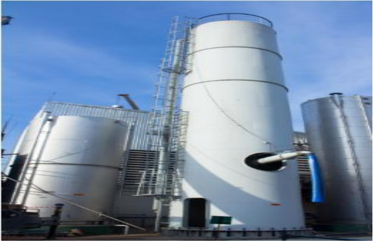
Figure 4.2.2 A silo or spent grain hopper
