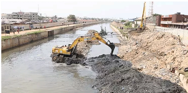
Fig. 12. Dredging of the Odaw river. Source: Graphic online
