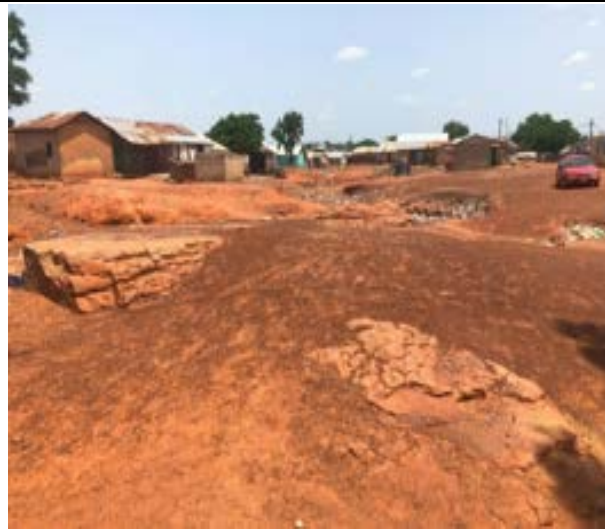
Figure 5.9 Rocky Terrain without drains
