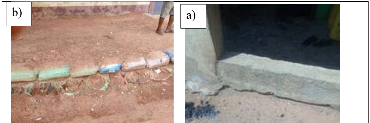
Figure 6.5 Images showing barrier construction
