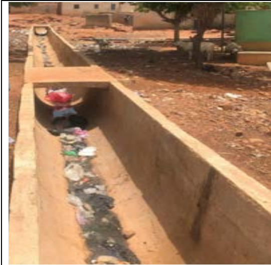
Figure 5.8 Constructed New Drain
