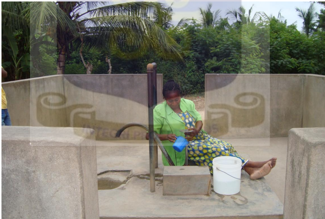
Plate 6-1: A caretaker at Worakesse Habitat doping the borehole with a foot pump with water to create the required pressure in the system for water abstraction.
