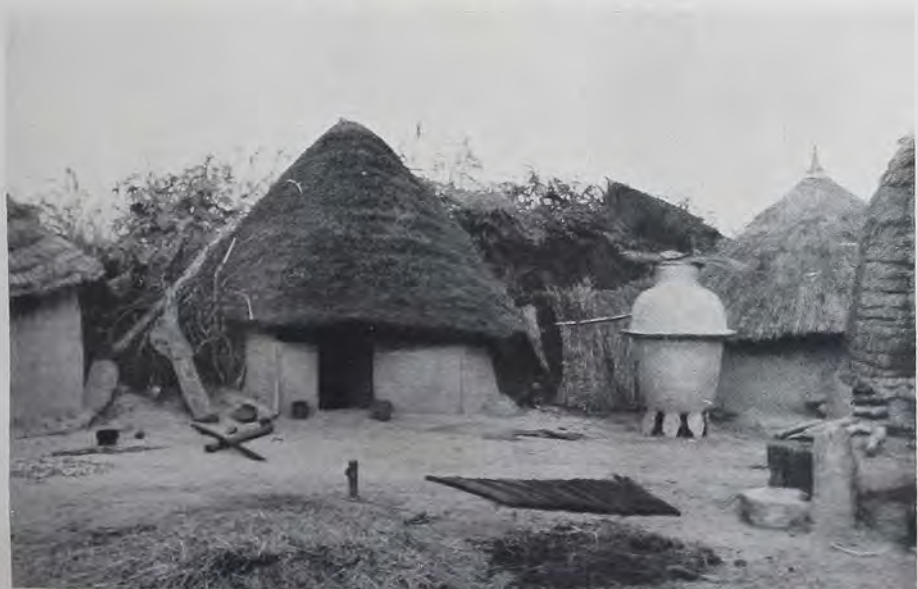
A family compound in the Pagan country near Zonkwa, Northern Nigeria. The roof of the dwelling-house in the centre is asymmetrical, with the apex towards the rear. This draws smoke away from the front room and provides a loft for storing firewood and other goods. The clay granary is supported on stone pillars to keep out white ants. The building behind the granary is used as a goat shed, and its doorway is barred by wooden logs behind upright stones.
