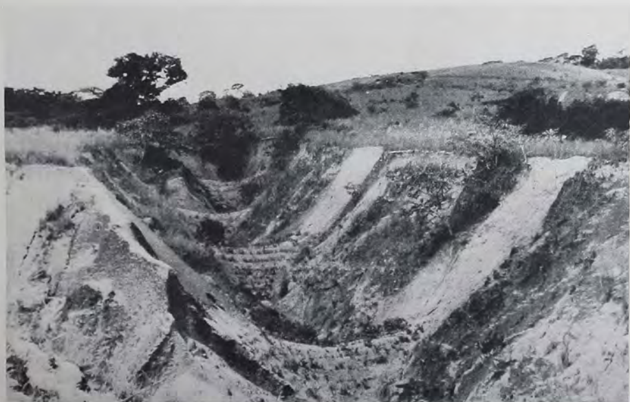
Gully erosion near Udi, Eastern Province, Nigeria. The gully in the centre is being checked by weirs
