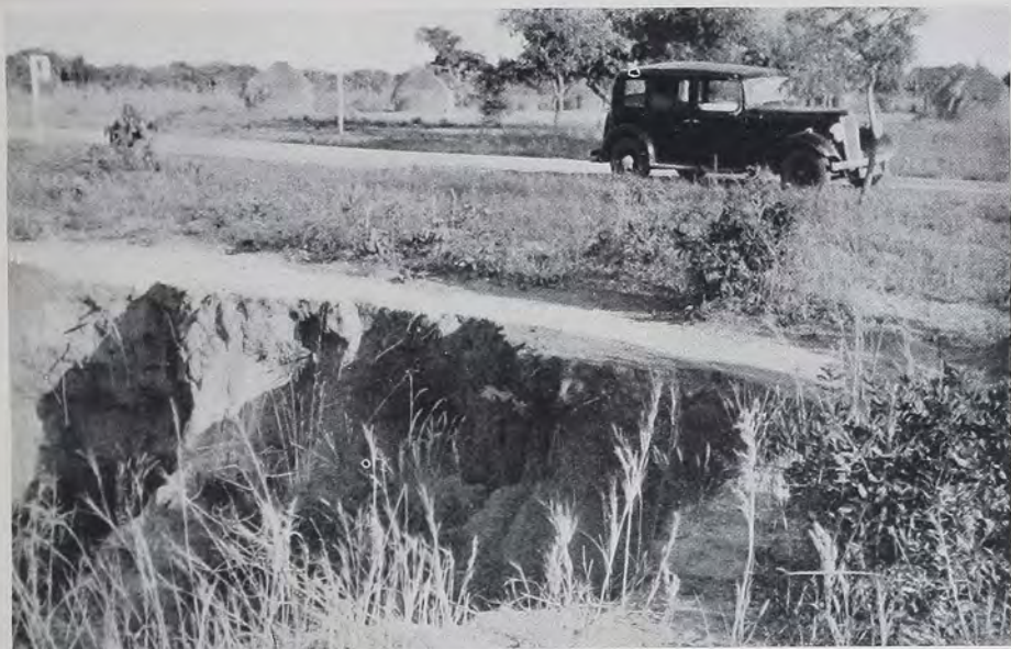
Gully erosion approaching main road near Zaria, Northern Nigeria
