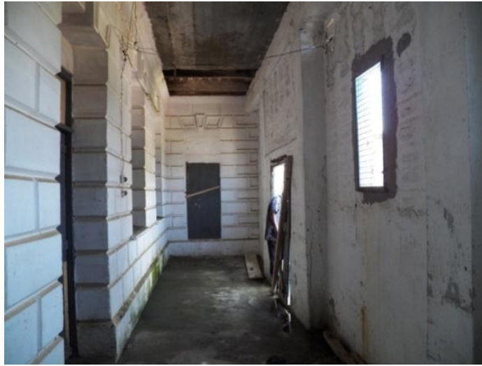
Plate 16: Concrete slabs introduced to support the wooden first floor slab
