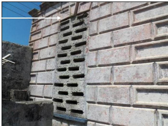
Plate 9: An altered opening showing a capstone which prominently features on door and window openings (Source: Author)
