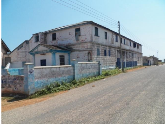
Plate 4: View of Northern façade at present ( Source: Author )
