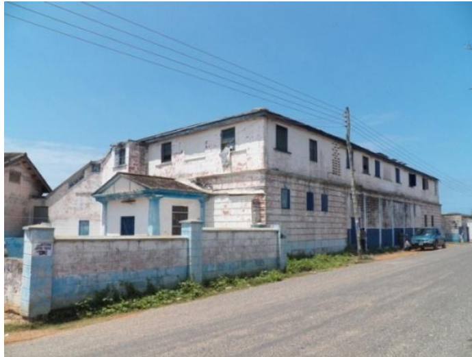
Plate 12: Northern and Eastern façades of the building showing alterations to the building for use by Pitman's College ( Source: Author )
