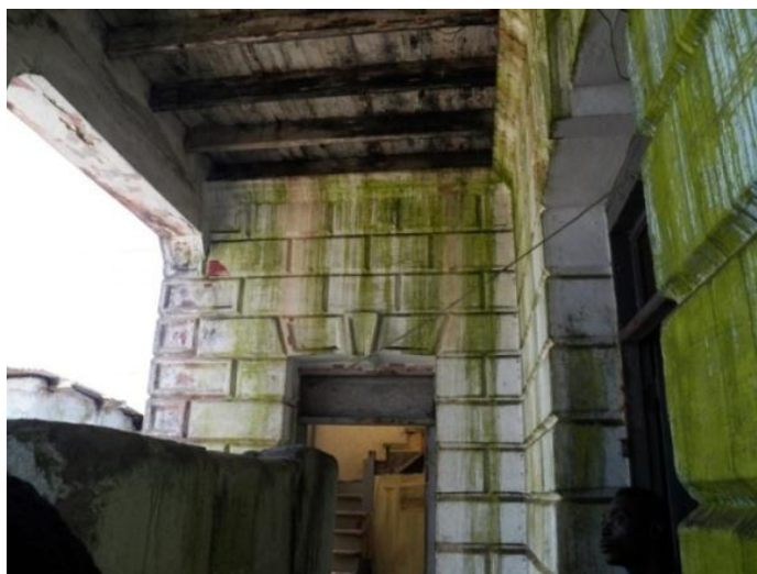
Plate 15: Effects of the prevailing climate on the building ( Source: Author )
