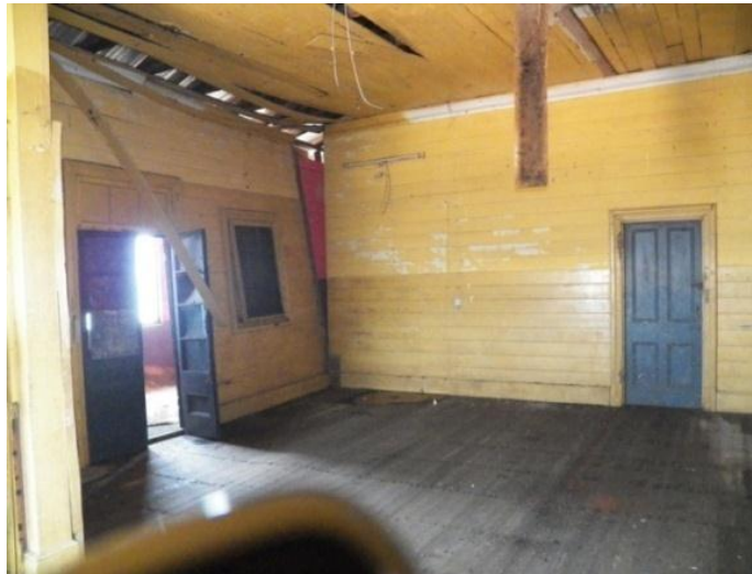
Plate 10: Wooden floor and partitions on the first floor ( Source: Author )
