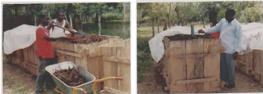
Plate 3.2: Building Compost Piles in Boxes Plate3.3: PVC Pipe ‡ Inserted into Pile to
