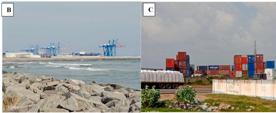
Plates B and C. New port terminal at Tema Port, and a container terminal infrastructure along the coast of Ghana. Photo credit: Richard Takyi.
