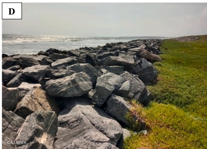
Plate D. Example of coastal defence structure along the Sakumono – Tema beach road in the Greater Accra Region of Ghana. Photo credit: Richard Takyi.
